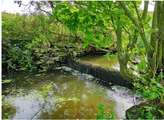
Weir restricting fish movement
