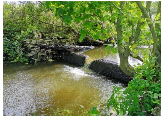
Weir after 'notching' to ease access
